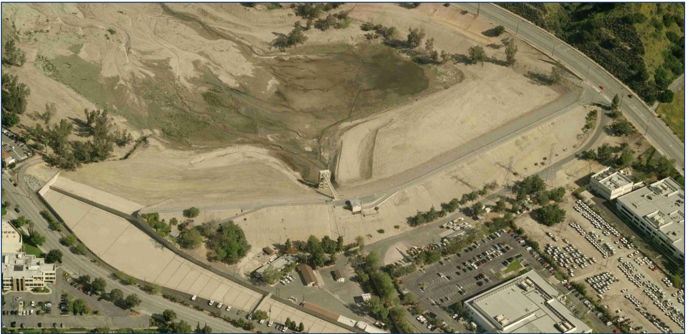
Figure 9-11 Eaton Wash Dam
