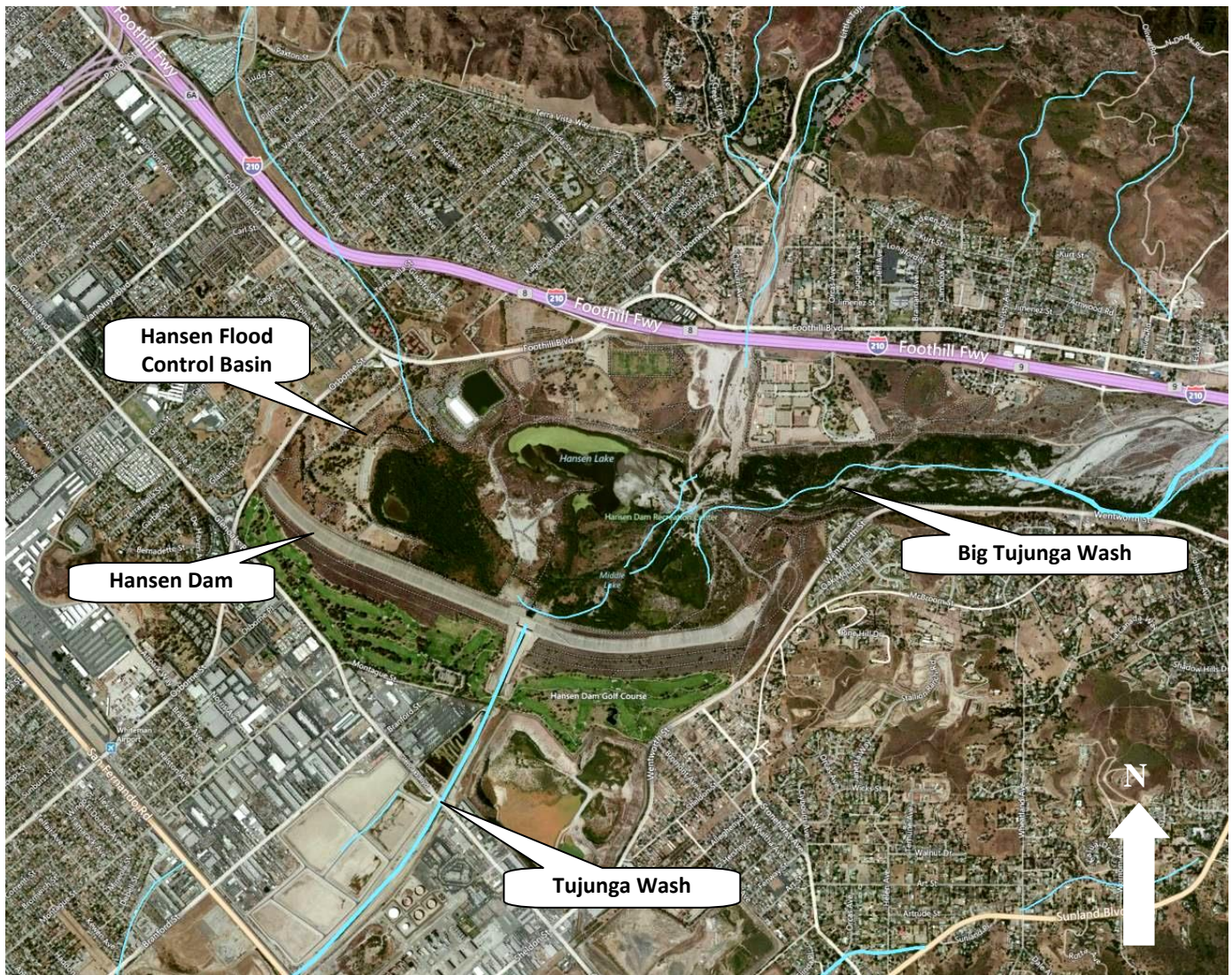
Figure 8-6 Hansen Flood Control Basin
