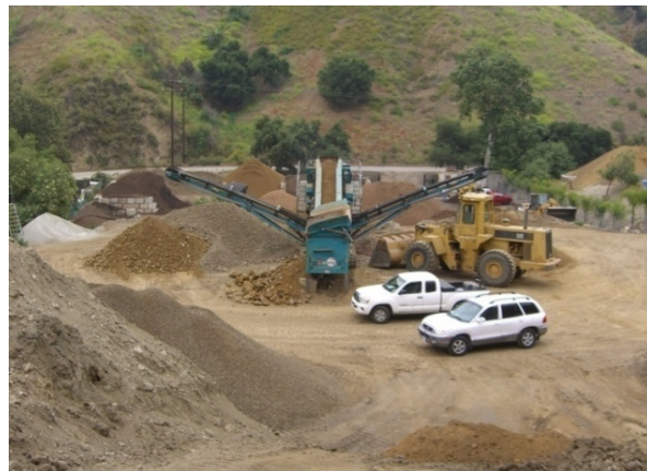
Photograph (right) – Power Double-Screen Operation
