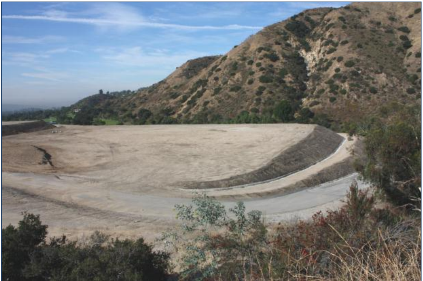
Figure 9-28 San Dimas SPS Looking Southwest
