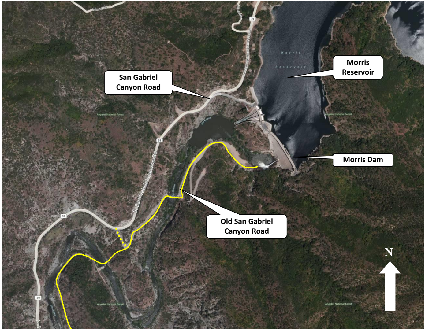
Figure 7-38 Morris Reservoir Access at Old San Gabriel Canyon Road
