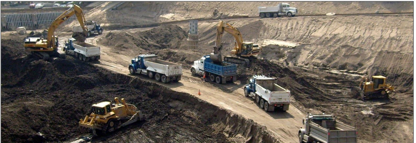
Figure 6-5 Excavation equipment loading single-dump trucks
