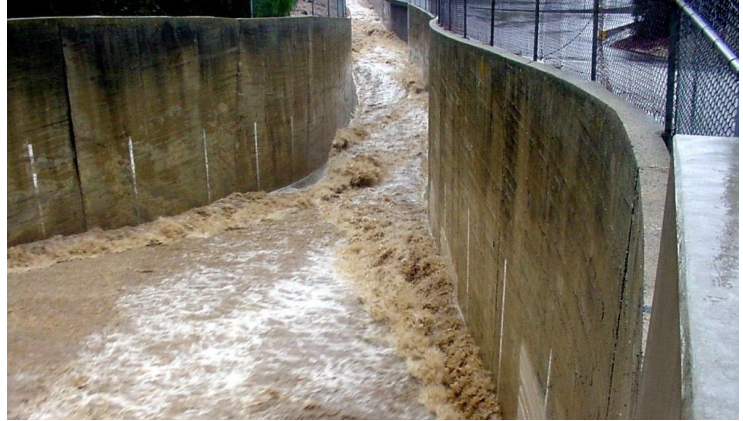
Figure 6-4 Channel flowing with sediment laden flow
