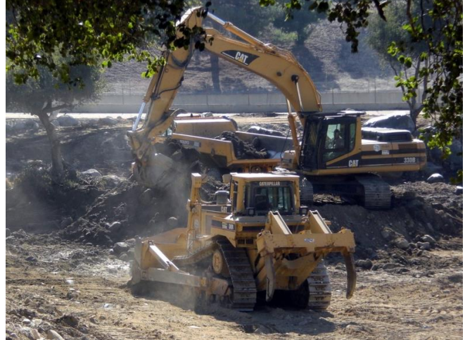
Figure 6-1 Equipment used during excavation
