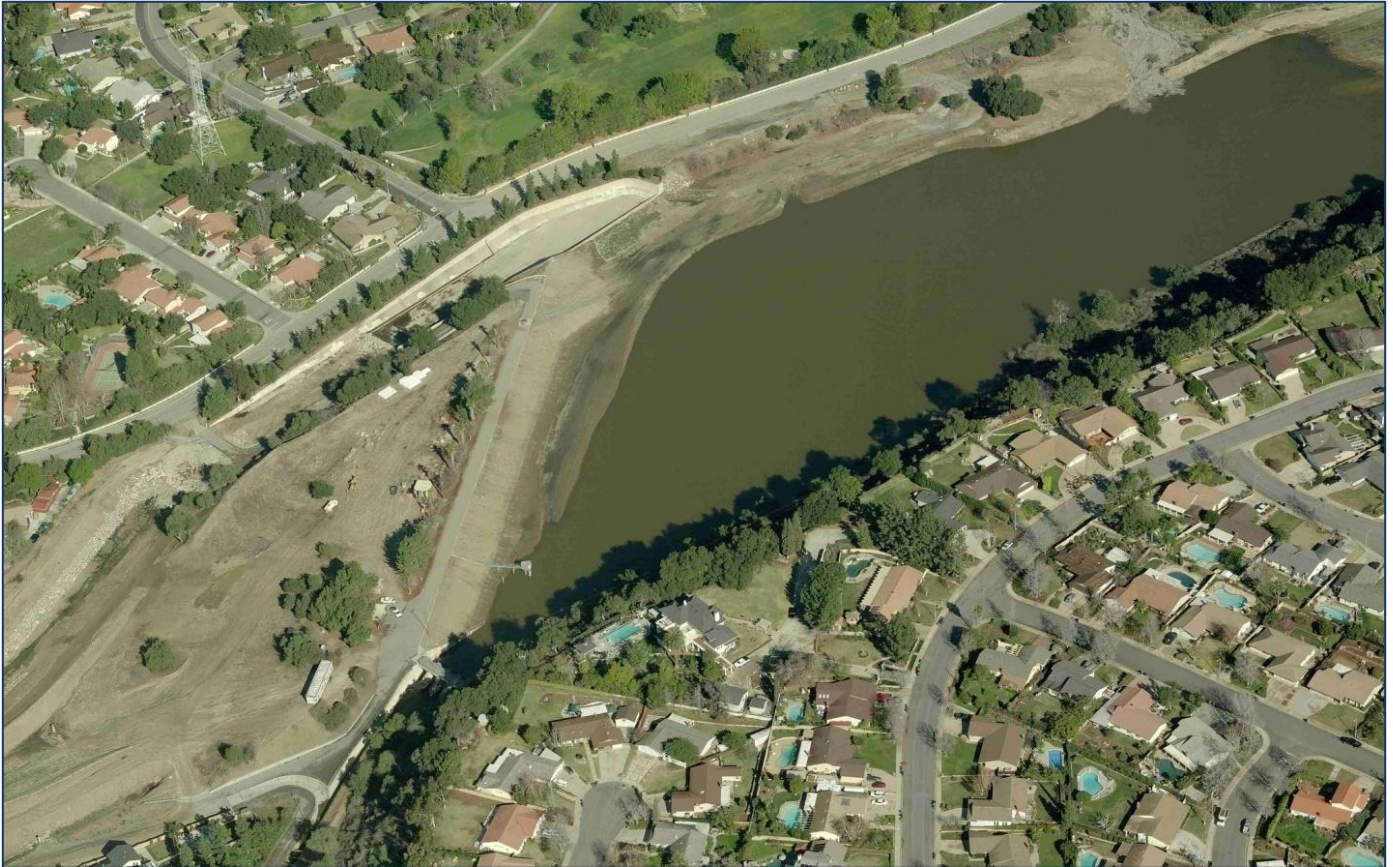
Figure 9-23 Puddingstone Diversion Dam
