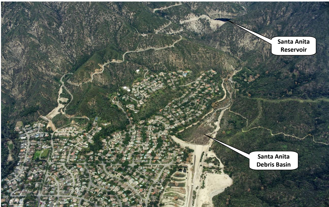
Figure 8-78 Santa Anita Debris Basin
