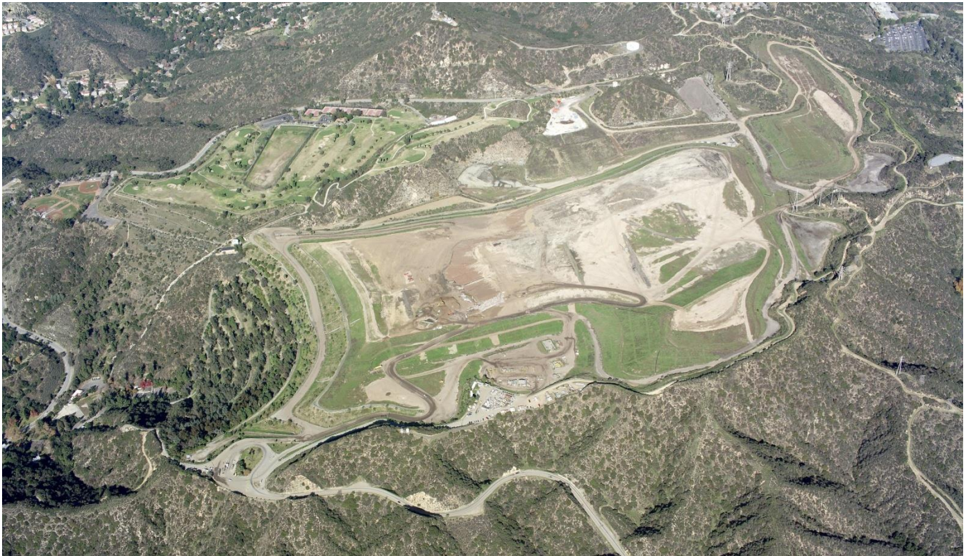
Figure 6-20 Scholl Canyon Landfill
