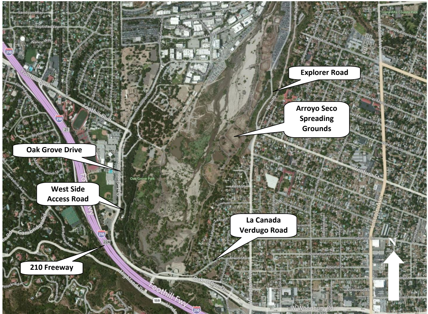
Figure 8-26 Devil’s Gate Dam and Vicinity
