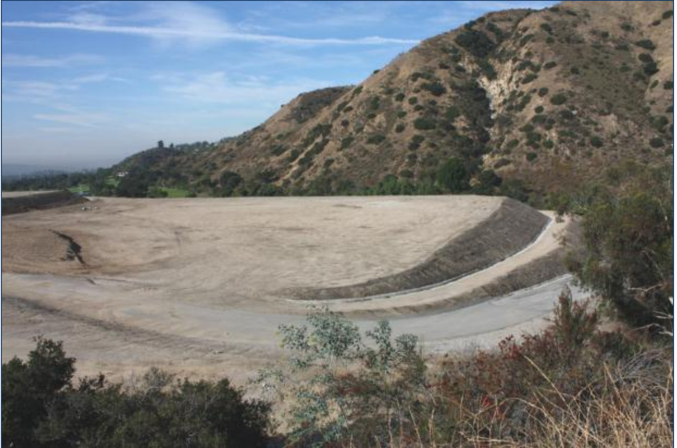
Figure 8-62 San Dimas SPS Looking Southwest
