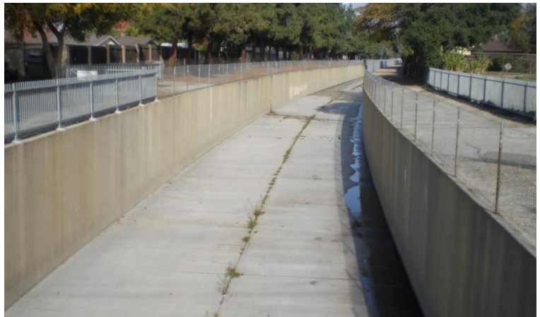
Figure 6-6 Typical Rectangular Channel
