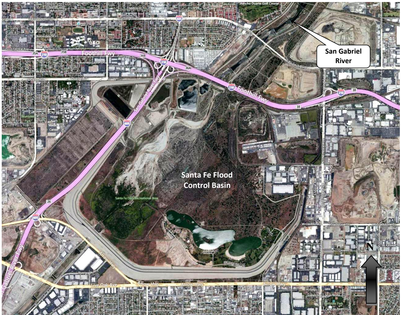
Figure 7-40 Santa Fe Flood Control Basin Aerial
