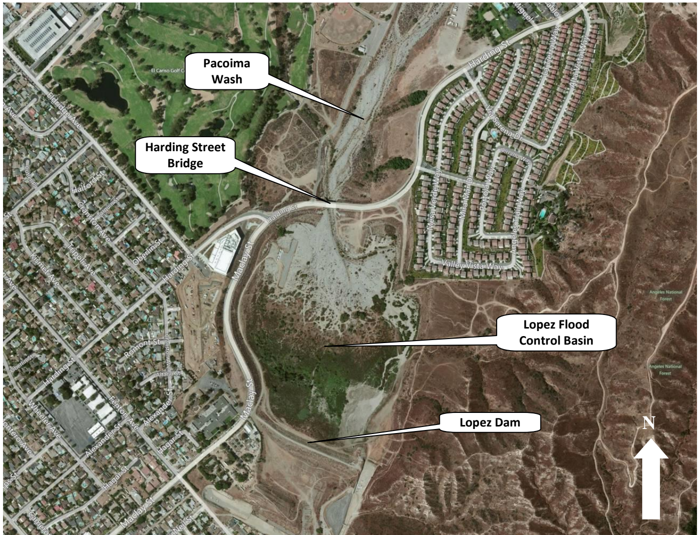
Figure 8-33 Lopez Flood Control Basin
