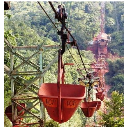
Figure 6-10 Cable bucket system
