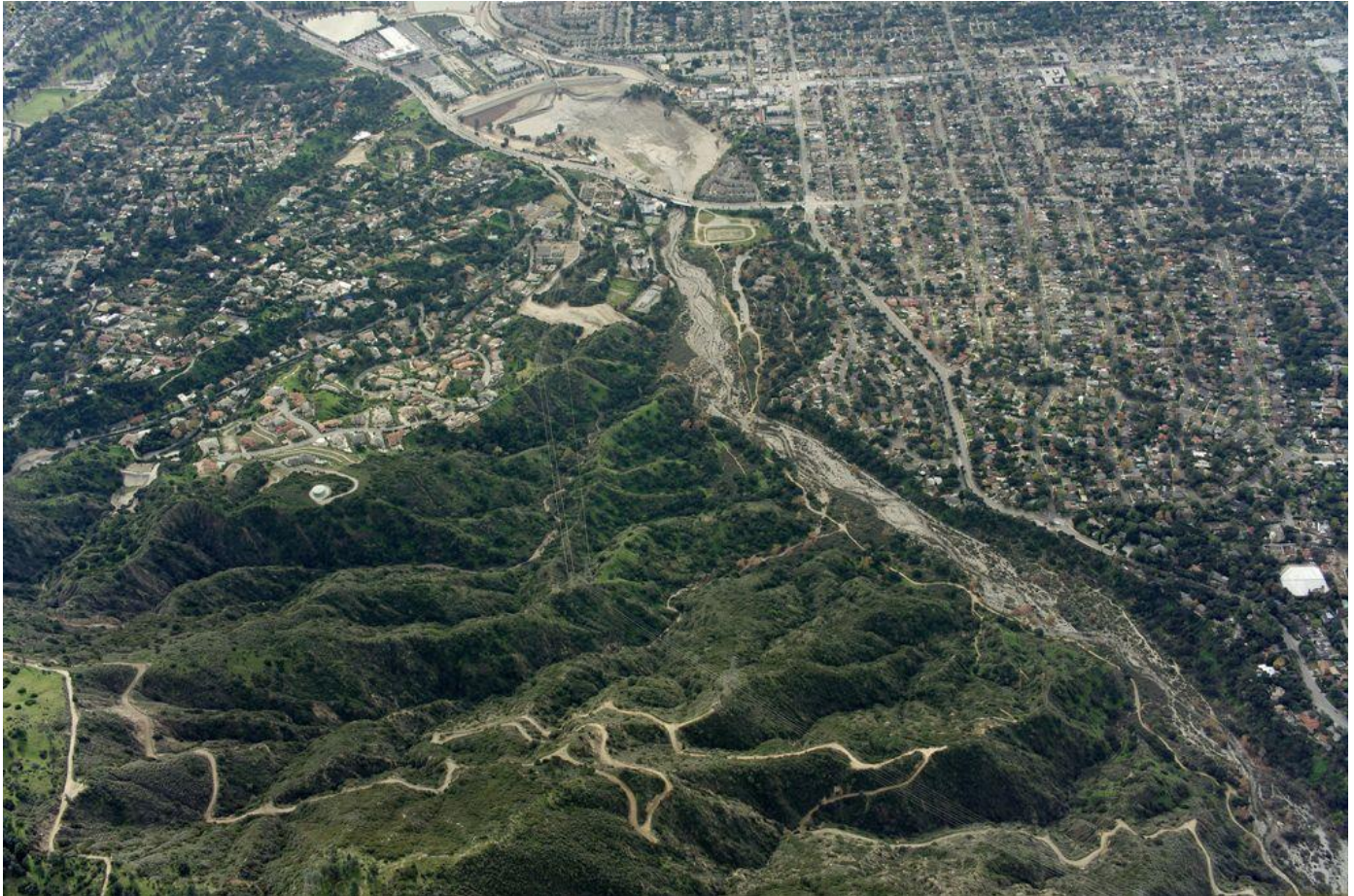
Figure 9-13 Eaton Wash Reservoir Topography
